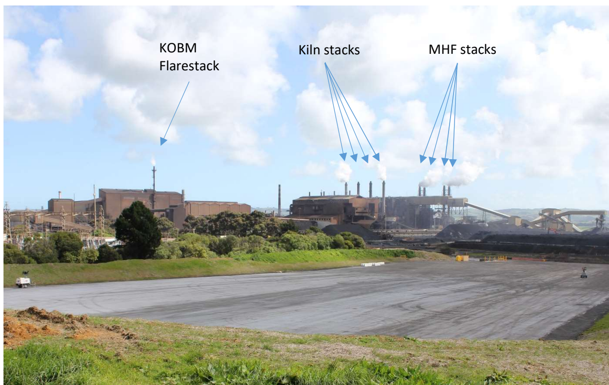
Figure 3.2: Image of Steel Mill showing MHF stacks, Kiln stacks and the KOBM Flarestack
