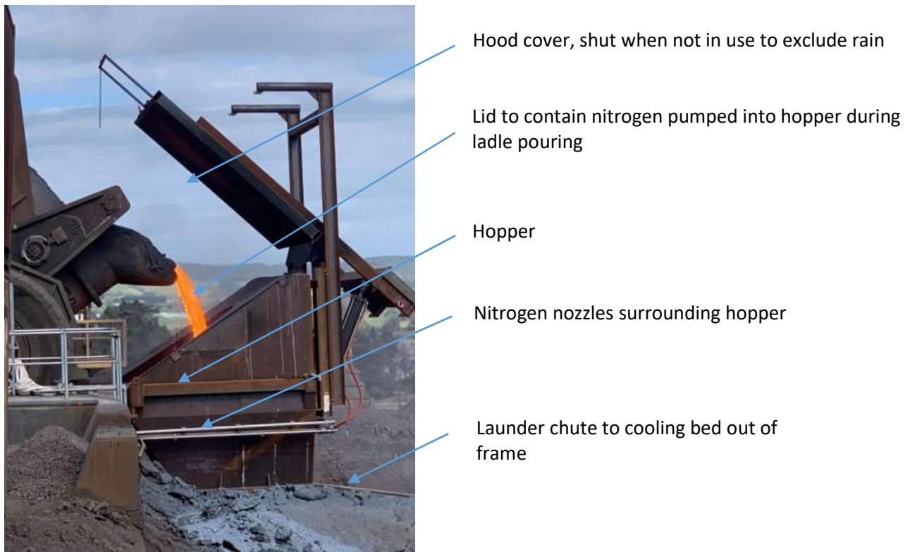
Figure 8.1: Molten iron poured to the fume suppression system
